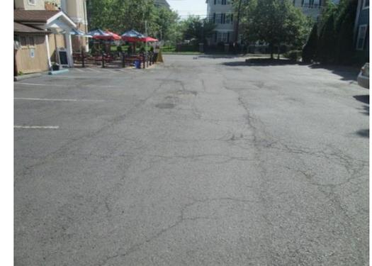
The parking lot drains to the roadway. Parking spaces can be replaced with porous asphalt to infiltrate stormwater. Pervious concrete can be installed to capture roof runoff draining onto the sidewalk on the west side of the building. A preliminary soil assessment suggests that the existing soils have suitable drainage characteristics for green infrastructure.
