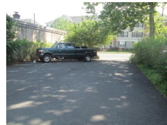
A rain garden can be installed to capture roof runoff from the disconnected downspouts in the gazebo area. The parking lot and driveway slope toward the road. Parking spots can be replaced with porous asphalt to infiltrate stormwater. A preliminary soil assessment suggests that the existing soils have suitable drainage characteristics for green infrastructure.
