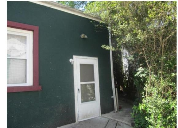
The building's downspouts are directly connected to the sewer system. Downspouts can be disconnected into planter boxes to treat the roof runoff before flowing into the street's drainage system. A preliminary soil assessment suggests that the existing soils have suitable drainage characteristics for green infrastructure.
