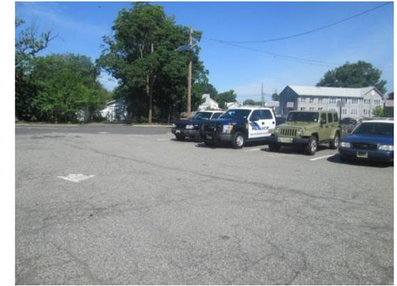
The parking lot slopes toward the building, down the driveway, and into the street. Parking spots can be replaced with porous asphalt to infiltrate stormwater. A preliminary soil assessment suggests that the existing soils have suitable drainage characteristics for green infrastructure.
