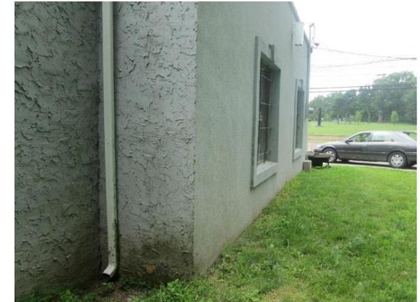
Stormwater from this site flows from the paved parking lot, and from the roof through disconnected downspouts. The downspouts can be redirected to infiltrate into the turf grass, and the parking spaces can be converted into pervious pavement to capture runoff. The gravel area should remain as it is partially pervious. A preliminary soil assessment suggests that more soil testing would be required before determining the soil's suitability for green infrastructure.
