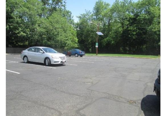
The apartment complex has large areas of pavement for parking that drain to catch basins. Portions of the parking lot can be replaced with porous asphalt to capture and infiltrate stormwater. Bioretention systems can be installed around the apartments to capture and treat roof runoff. A preliminary soil assessment suggests that further testing will need to be done to determine if it has suitable drainage characteristics for green infrastructure.
