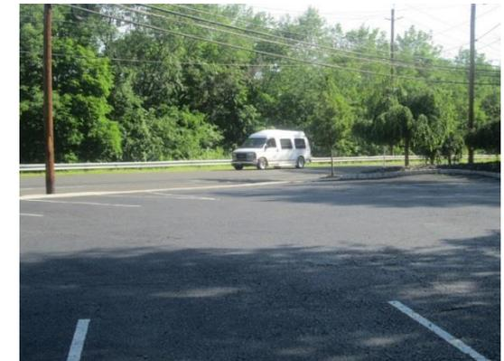
The paved areas are pitched to the street. Parking spaces on the west and northeast sides of the building can be replaced with pervious pavement. The west side can also capture rooftop runoff from existing downspouts. A preliminary soil assessment suggests that the existing soils have suitable drainage characteristics for green infrastructure.
